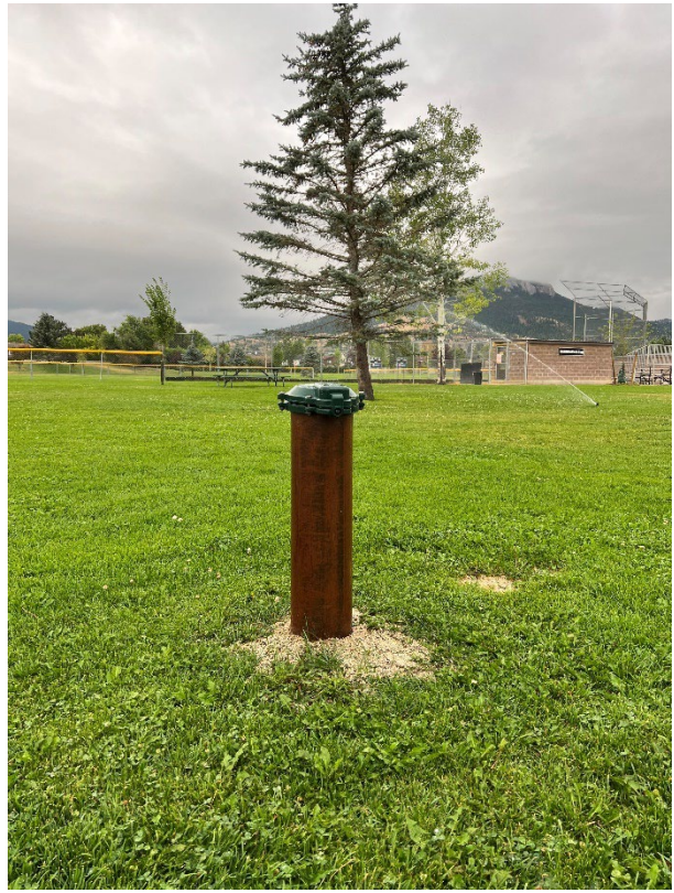
Figure 2: Image of Well Head
