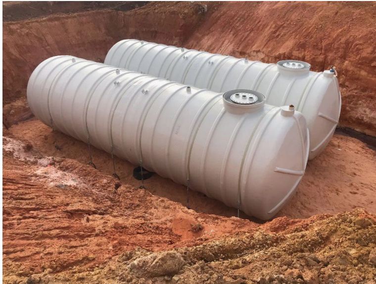
Figure 3: Underground Water Tanks
