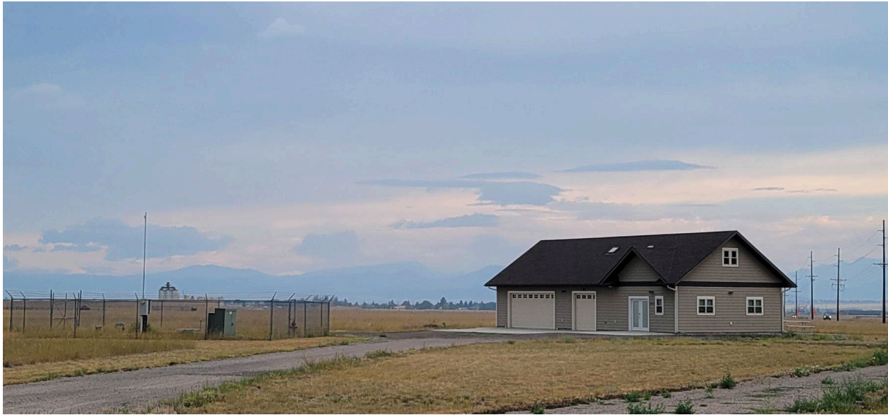
Figure 4: Well and Pumping Facilities Building
